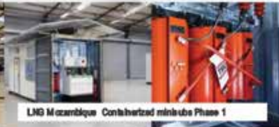
Containerized MCC & Specialised Wall Mounted VSD's - Delivered to Africa
